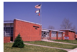
Madison is one of the schools that will undergo energy efficiency upgrades.
