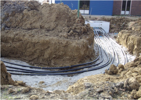
Preparation for a geothermal well field at Jackson
